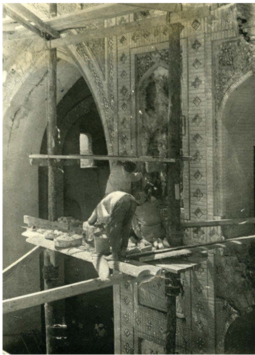
Figure 11.24: “Work on reinforcing the structure on the right-hand side of the mosque’s door, Anau, 1936”. Photo by Nikolai Mikhailovich Bachinskii. Archive of the Institute for the History of Material Culture, Russian Academy of Sciences.
